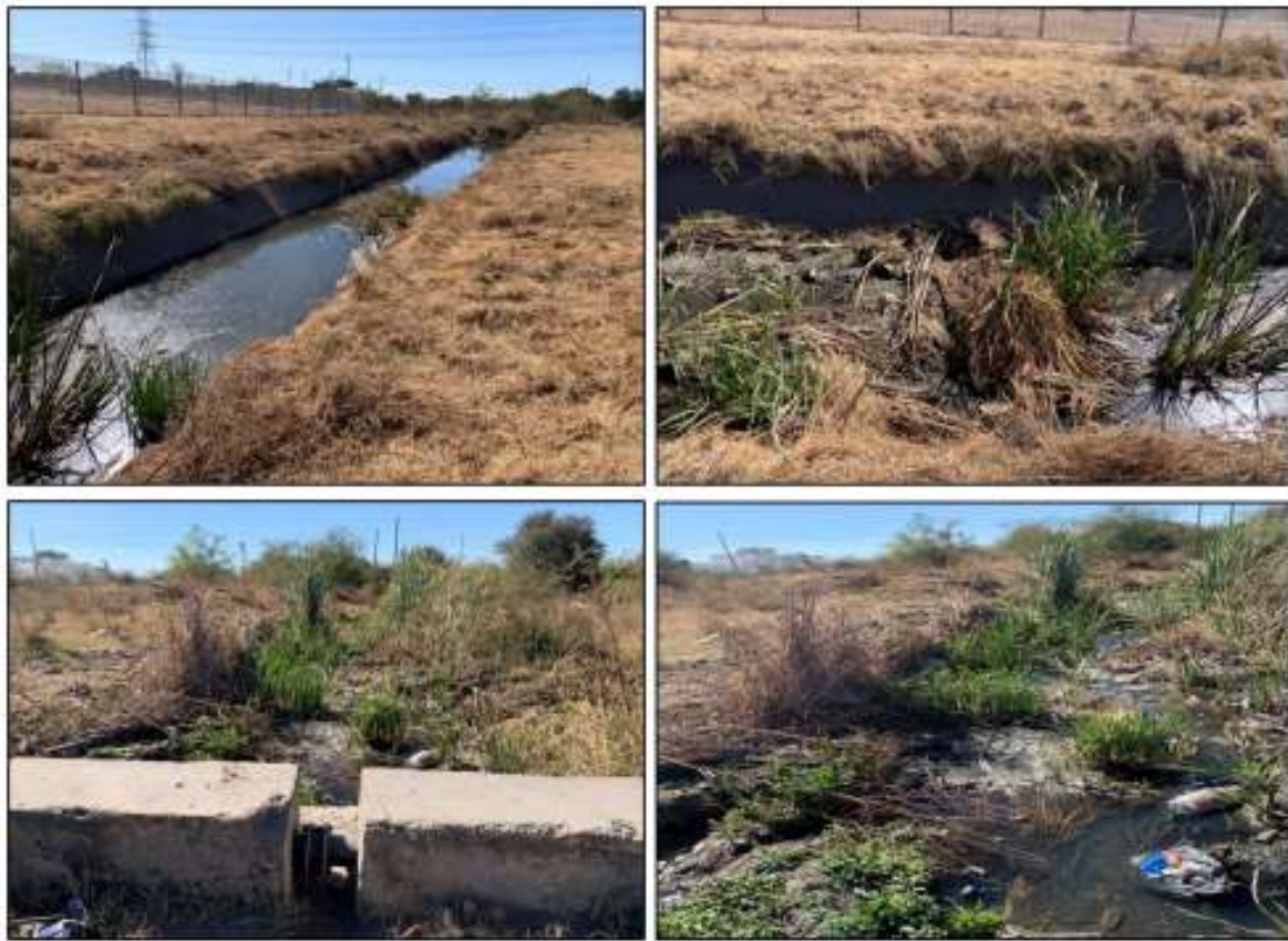
FIGURE 20 REPRESENTATIVE PHOTOGRAPHS OF THE ARTIFICIAL FEATURE (TOP) WHICH DRAIN INTO THE NORTH EASTERN CVB WETLAND (BOTTOM). THE ARTIFICIAL FEATURE HAS BEEN CHANNELLED BY MEANS OF CONCRETE EMBANKMENTS (SAS, 2024)
