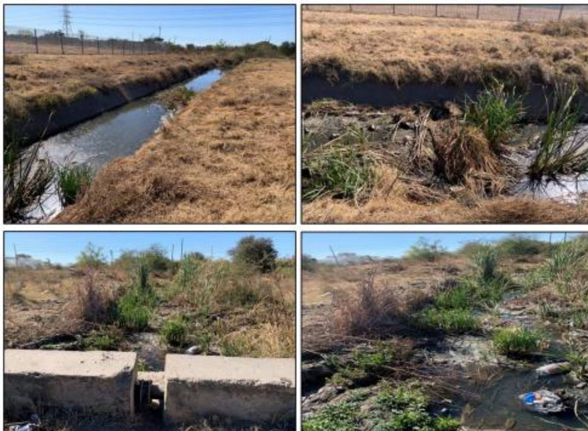
FIGURE 20 REPRESENTATIVE PHOTOGRAPHS OF THE ARTIFICIAL FEATURE (TOP) WHICH DRAIN INTO THE NORTH EASTERN CVB WETLAND (BOTTOM). THE ARTIFICIAL FEATURE HAS BEEN CHANNELISED BY MEANS OF CONCRETE EMBANKMENTS (SAS, 2024)
